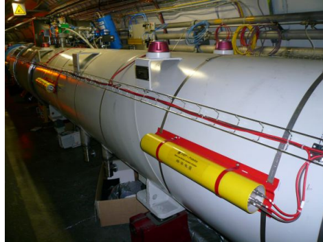
Fig. 1. An ionization chamber installed on the side of the magnet in the tunnel
