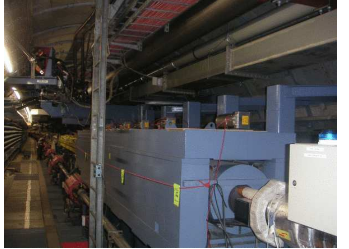
Fig. 8. Installation of beam loss detectors on top of the HERA proton beam dump.
