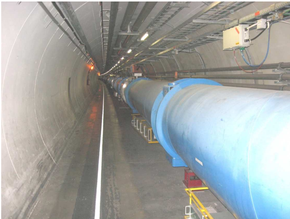
Fig.3.1.1: The LHC tunnel. Main Dipoles are blue, Main Quadrupoles – grey.
